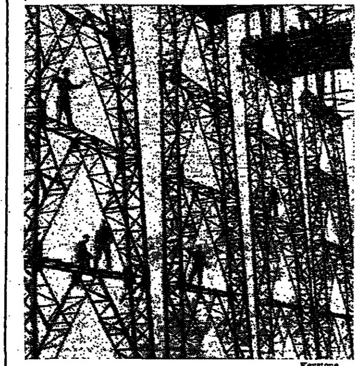
DESIGN FOR POWER—A new Soviet electric power plant at Inguri forms a pattern against a bright sky.
